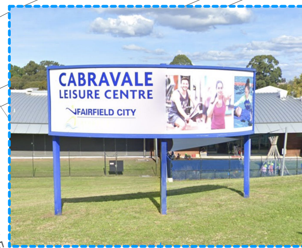
Existing signage to be removed
